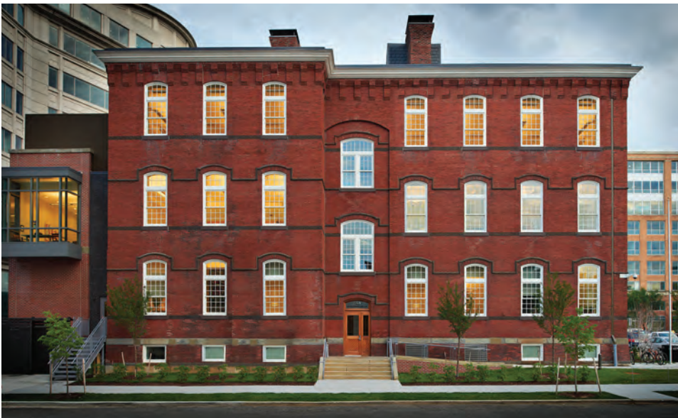
When specifying windows it is very important to take into consideration both rough and masonry openings.
