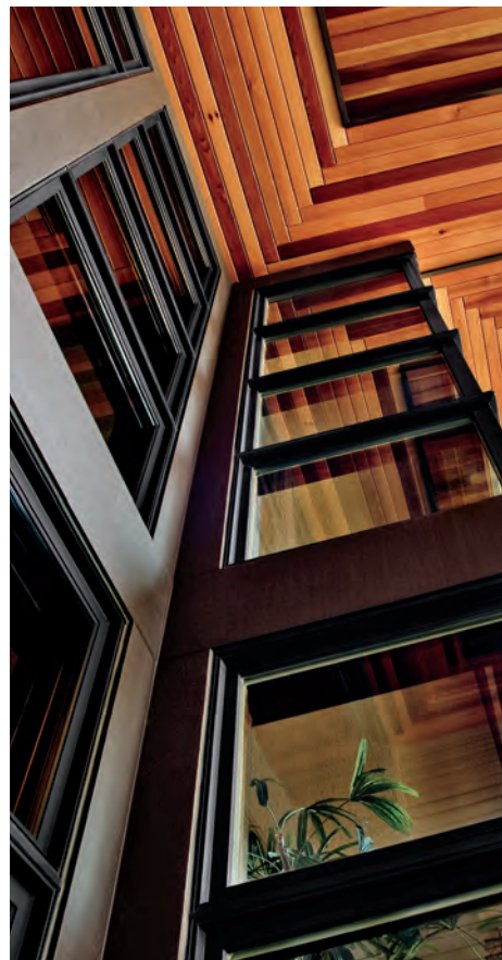
The frame description should include the window style and shape, both interior and exterior finishes, basic dimensions such as the thickness and depth of the frame, and the use of certified wood, if required.
