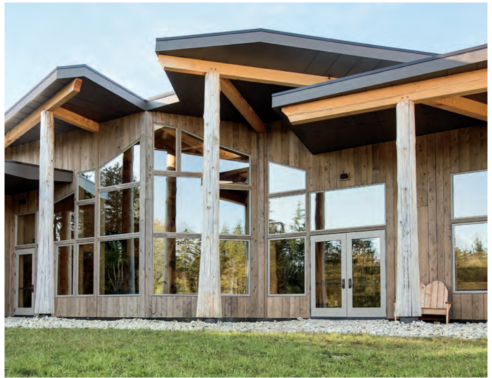
Mock-ups can provide installers an understanding of potential issues and causes of failures from "normal" or traditional installation techniques prior to assemblies being constructed on the actual building.
