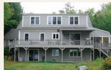
Before the remodel.
